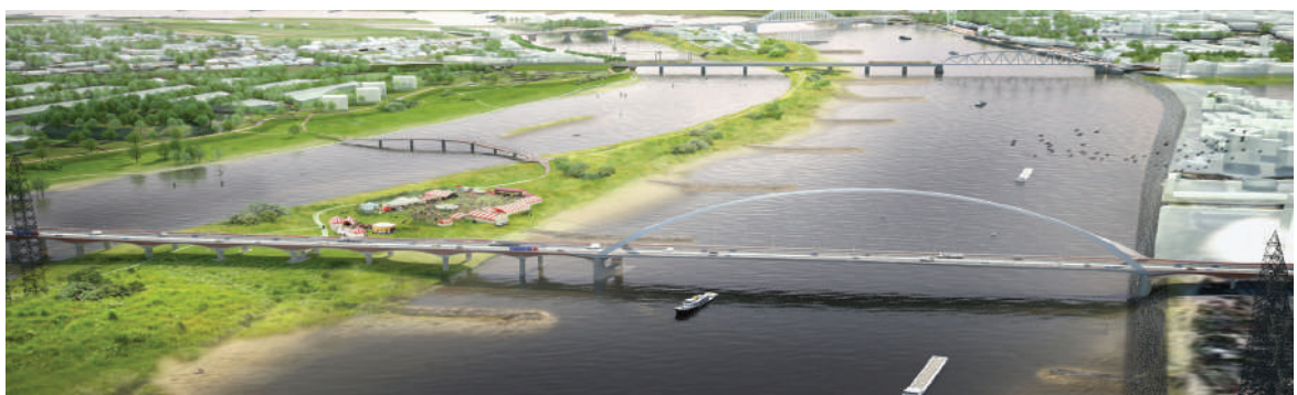
Figure 19 | Secondary channel and island developed as part of the Room for the River program near Nijmegen
