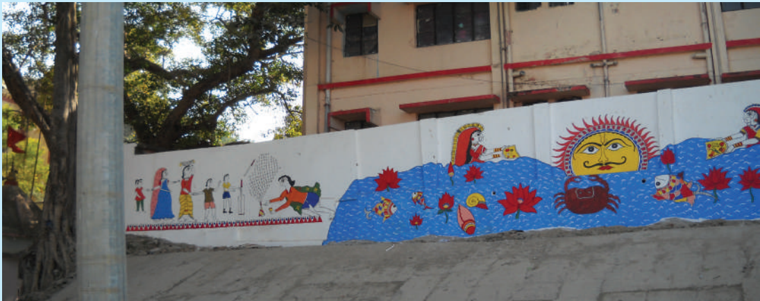
Figure 15 | Embankment walls along riverfront to protect built spaces in the city
